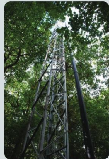
▲ Tower supporting black plastic pipe from which carbon dioxide is released
